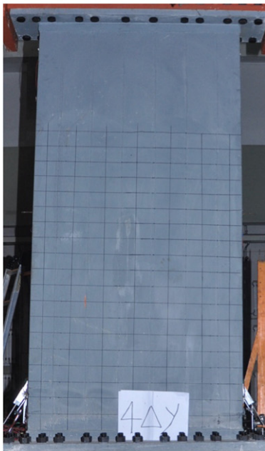
(c) Failure photo
