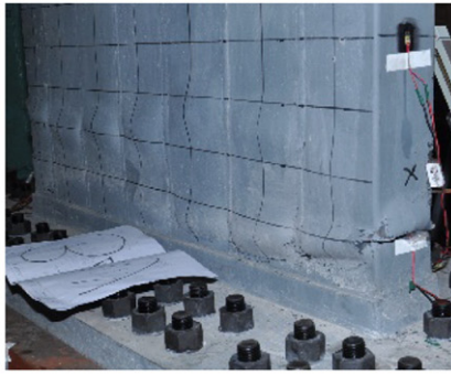
(a) Severe buckling and concrete crushing
