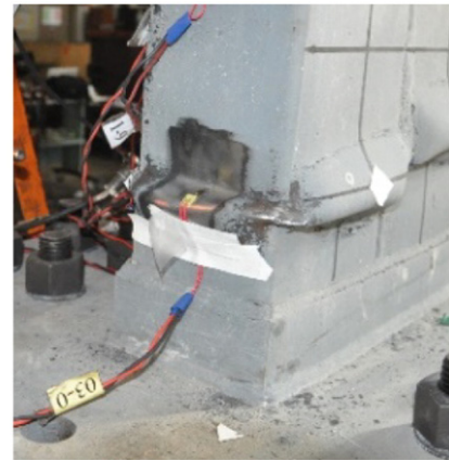
(a) Local buckling
