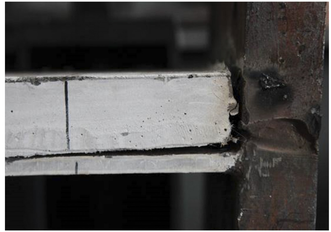
Fig. 11. Rupture of reinforcement–end plate welding
