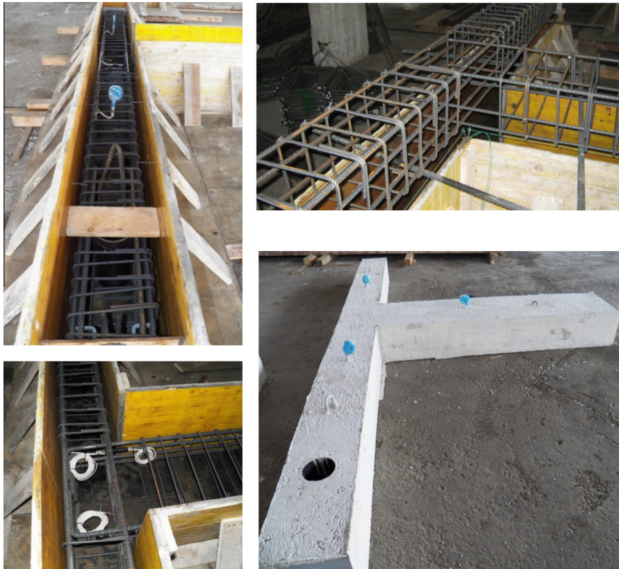
Fig. 2. Construction of specimens.
