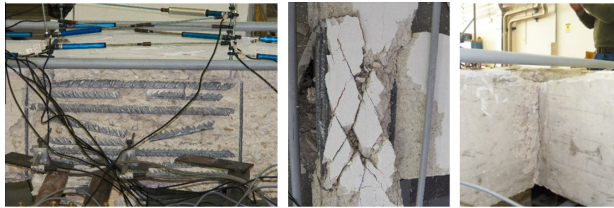
Fig. 8. Final damage state: joint panel and beam–joint interface – Test #1.
