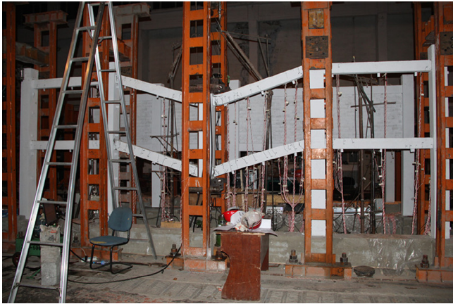
Fig. 9. Failure mode of the bare frame at the end of the test.
