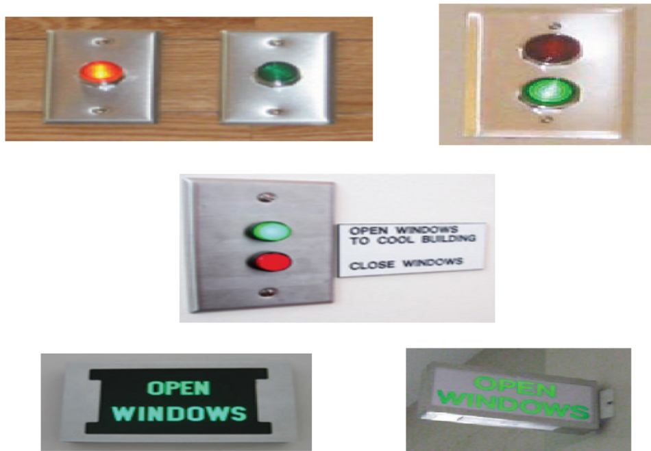
Fig. 3. Signal Interface Types* [53] *(top) unlabeled open/close indicator lights, (middle) labeled open/close indicator lights, (bottom) on/off lighted open signals.
