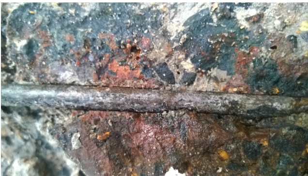
Fig. 8. Corroded rebar after electrochemical experiment.
