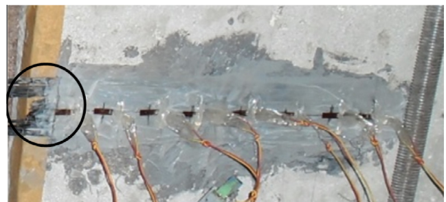
Fig. 10. Failure of a test specimen with the rupture of FRP sheet.
