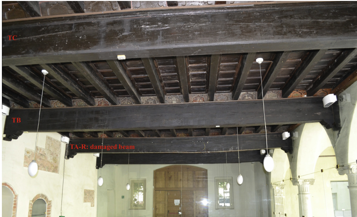
Fig. 3. Wooden floor of "Palazzo Calini ai Fiumi" before the repair (Brescia – Italy).
