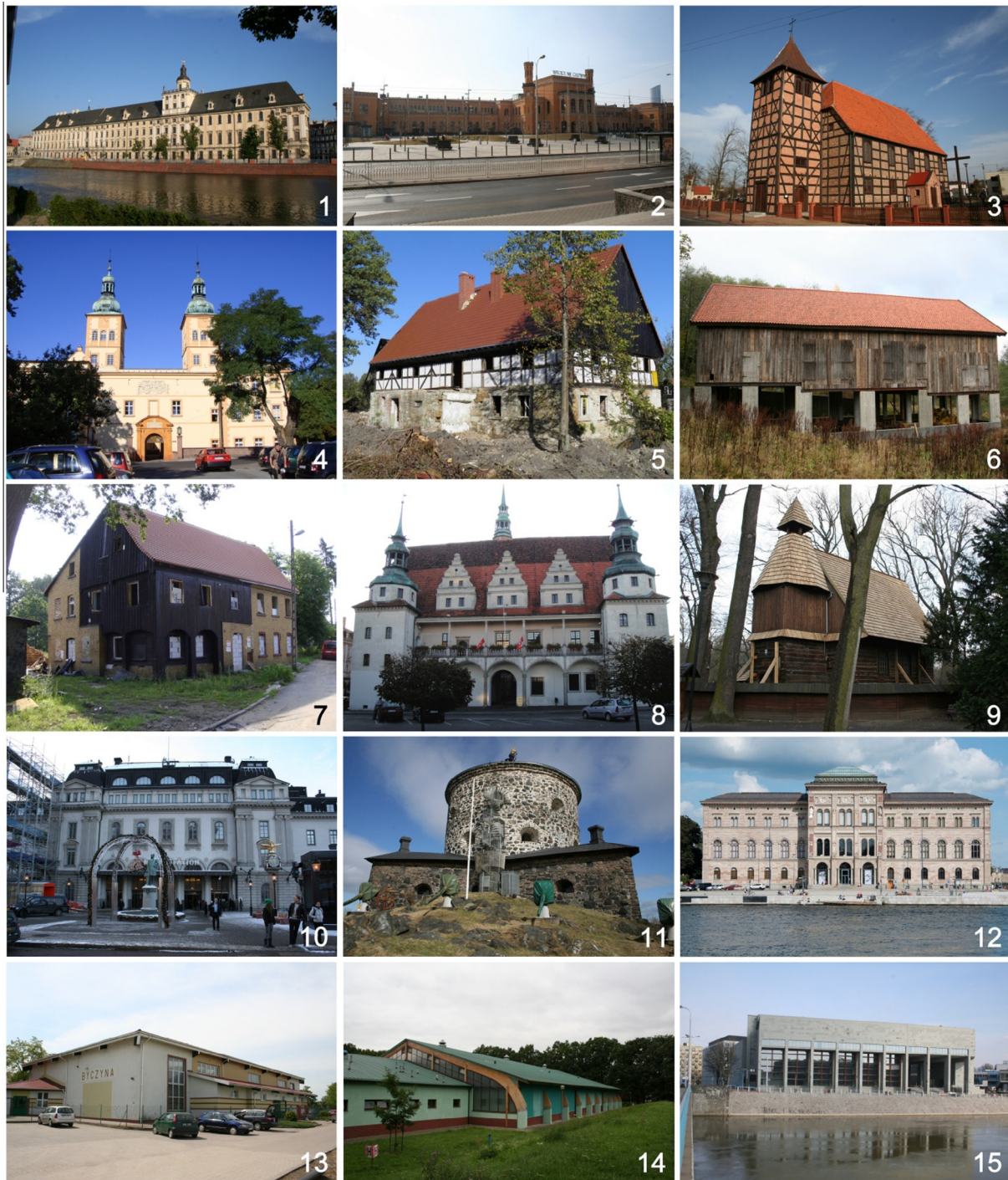
Fig. 5. Buildings for which drilling resistance tests have been carried out (numbered in accordance with descriptions in the text and in Table 3).
