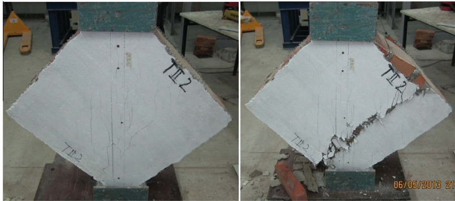
Fig. 5. TRM (TII) jacketed walls on both sides: (a) crack initiation along the compressed diagonal; (b) excessive cracking occurs and de-bonding.
