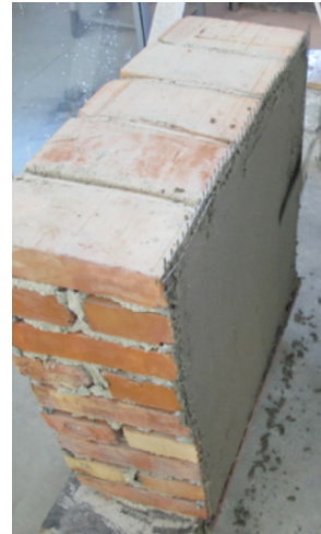
(a) Application of TRM strengthening to masonry walls
