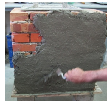
(c) Application of PP-FRM strengthening of masonry walls
