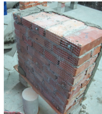
(b) Application of Ferrocement strengthening of masonry walls
