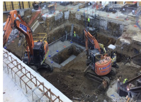
Construction site for case study B
