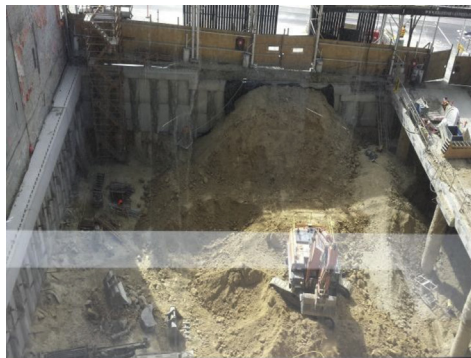
Construction site for case study A
