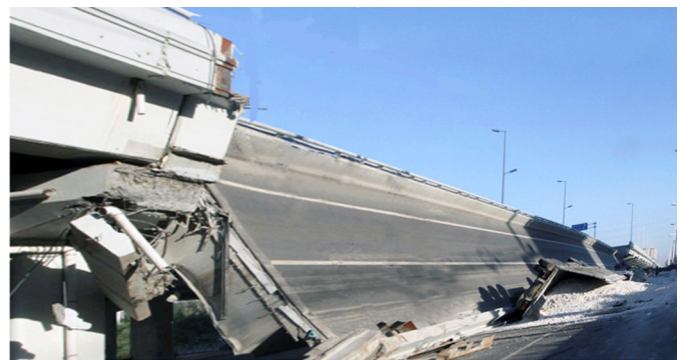
Fig. 5. Collapse scene of Yangmingtan Bridge (image courtesy of Xiaojiang Zhang)
