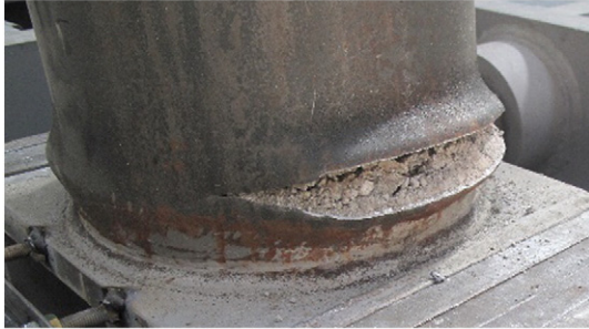
Fig. 13. Fracture of the steel tube during a cyclic test.
