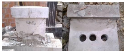
(a) Core drilling from wall specimens
