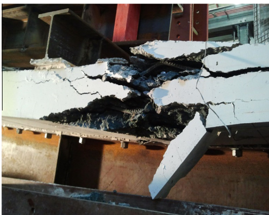
Fig. 17. Crushing of concrete slab and local buckling of rebar at mid-span.
