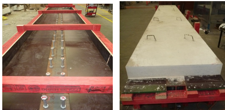
(a) SEBSCs on top flange (b) after concrete casting
