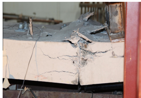
Fig. 19. Concrete cracking development of specimen CB2.
