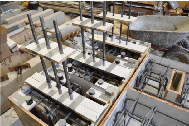
Fig. 7. Reinforcing cages and formwork for pullout specimens.
