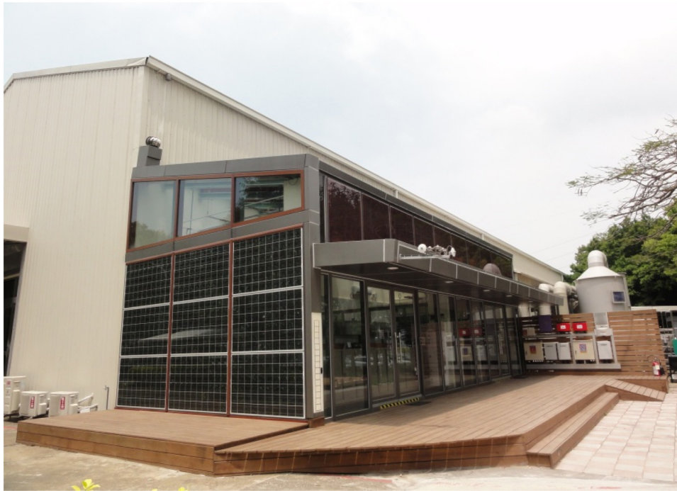
Fig. 3. The BIPV Experiment Demonstration House.
