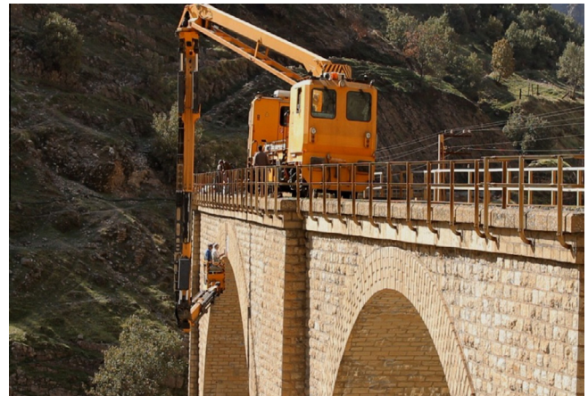
Fig. 5. DCDT placement on the keystone and the quarter point of span length.
