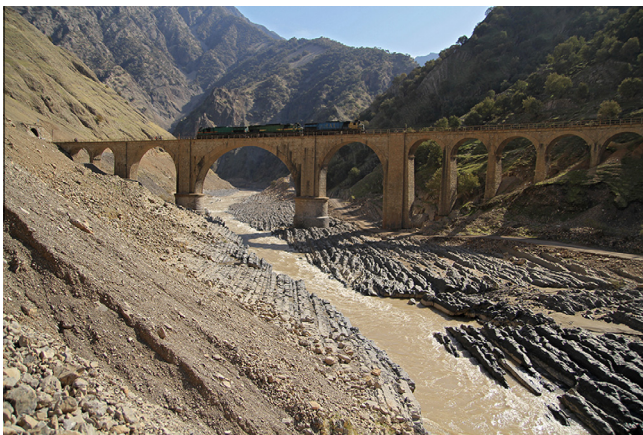
Fig. 2. Overall view of the bridge.
