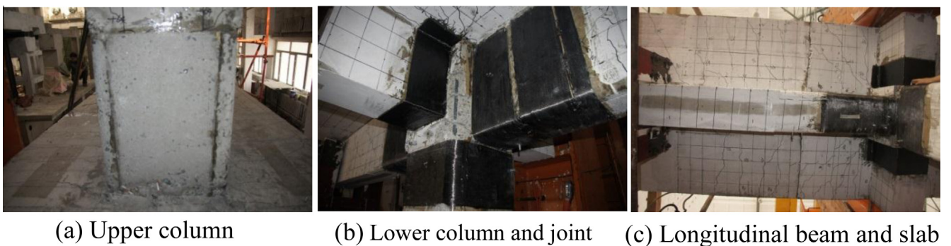
Fig. 10. Failure modes of specimen SCBW.
