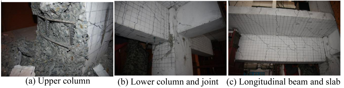
Fig. 7. Failure modes of specimen C.
