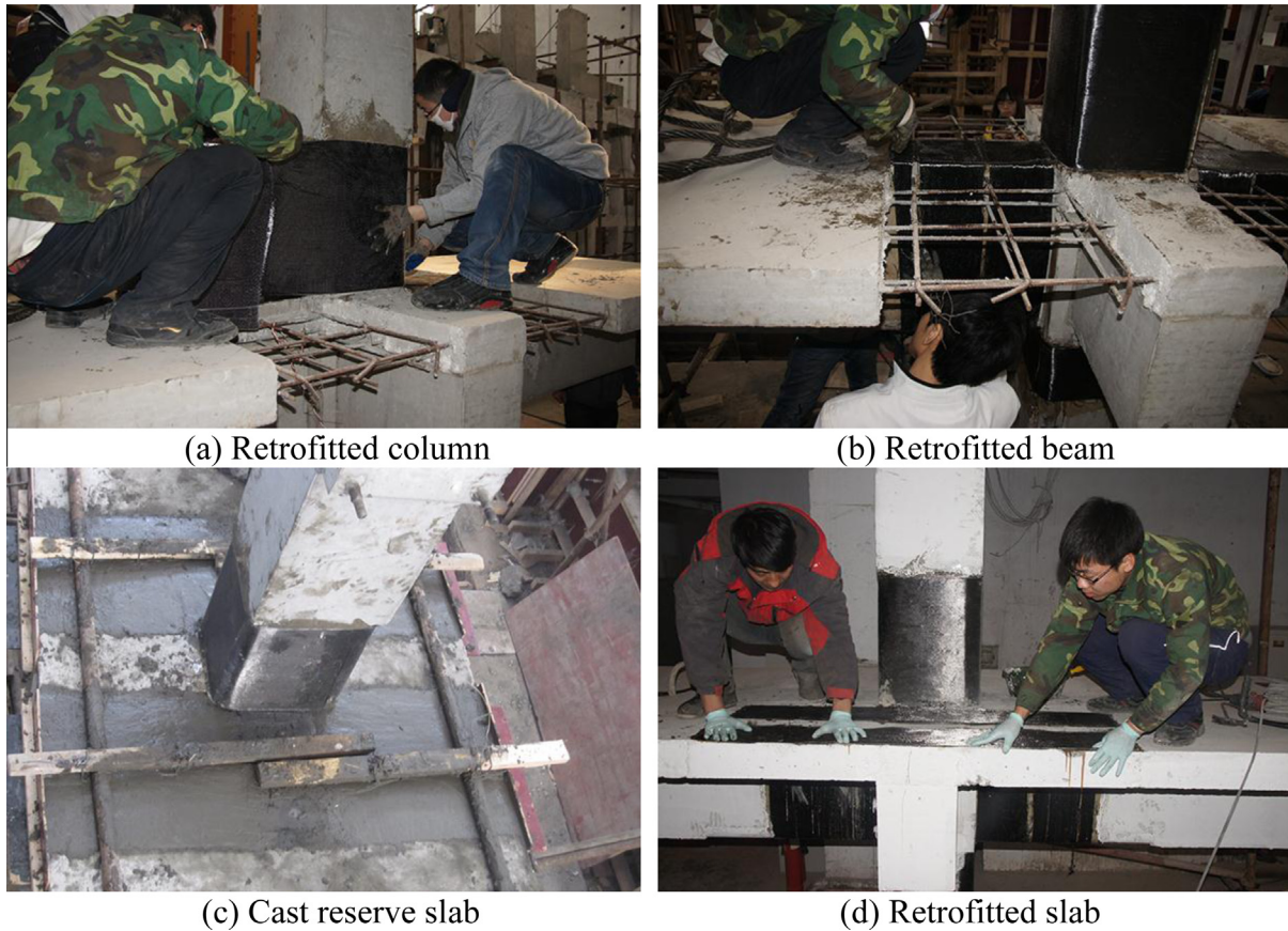
Fig. 3. Pictures showing retrofitted process of specimen SCBW.
