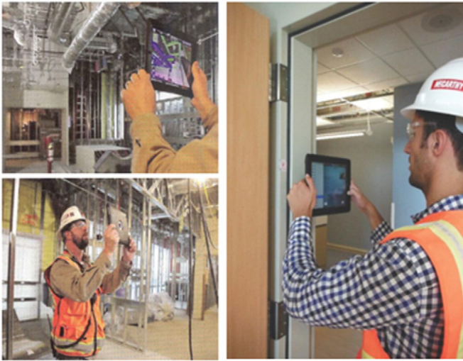
Fig. 3. Data acquisition and as-built status capturing using BIManywhere.
