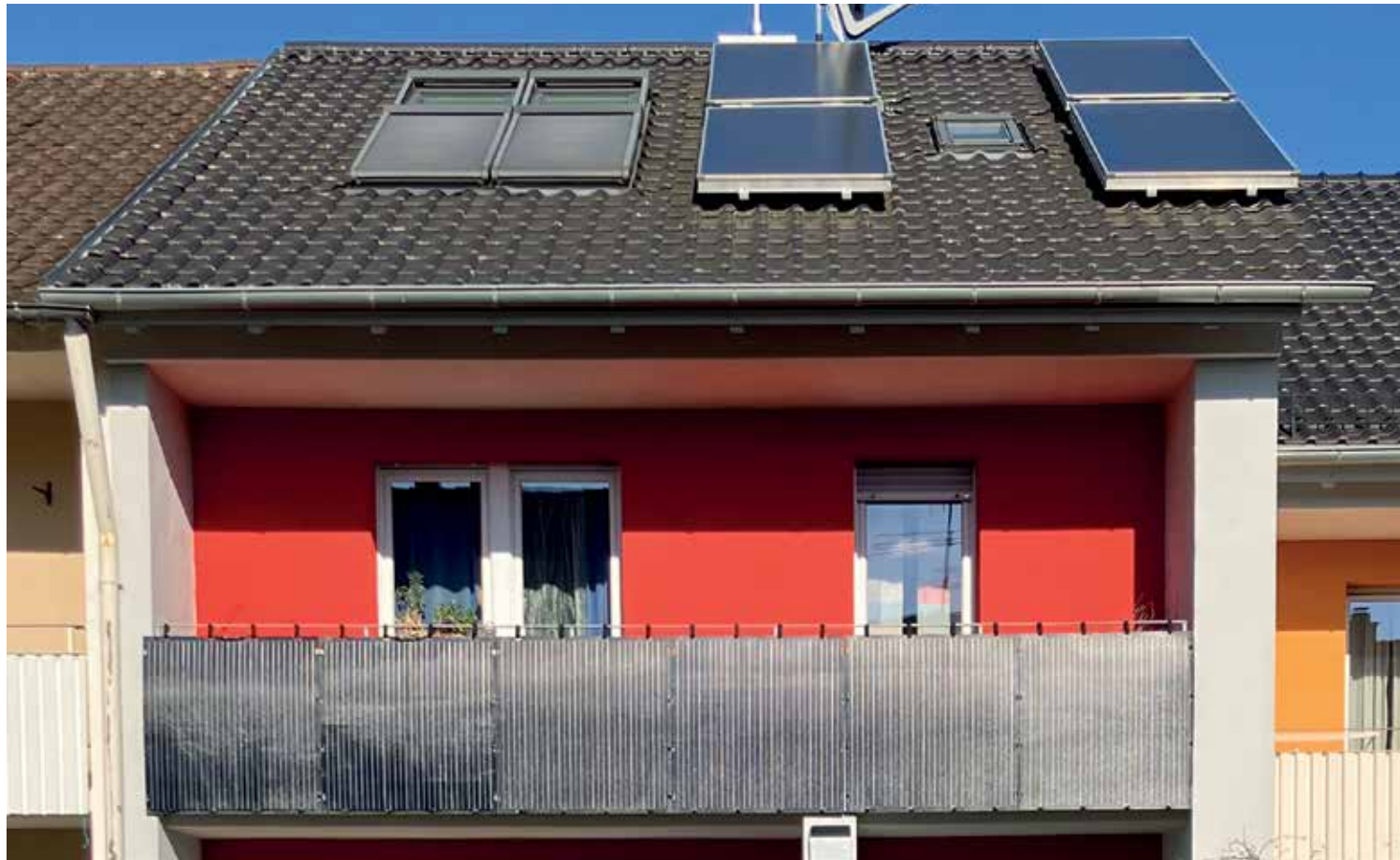
Figure 13.1. A balcony power plant – example from Germany (Source: Michael Waibel, 2023)
